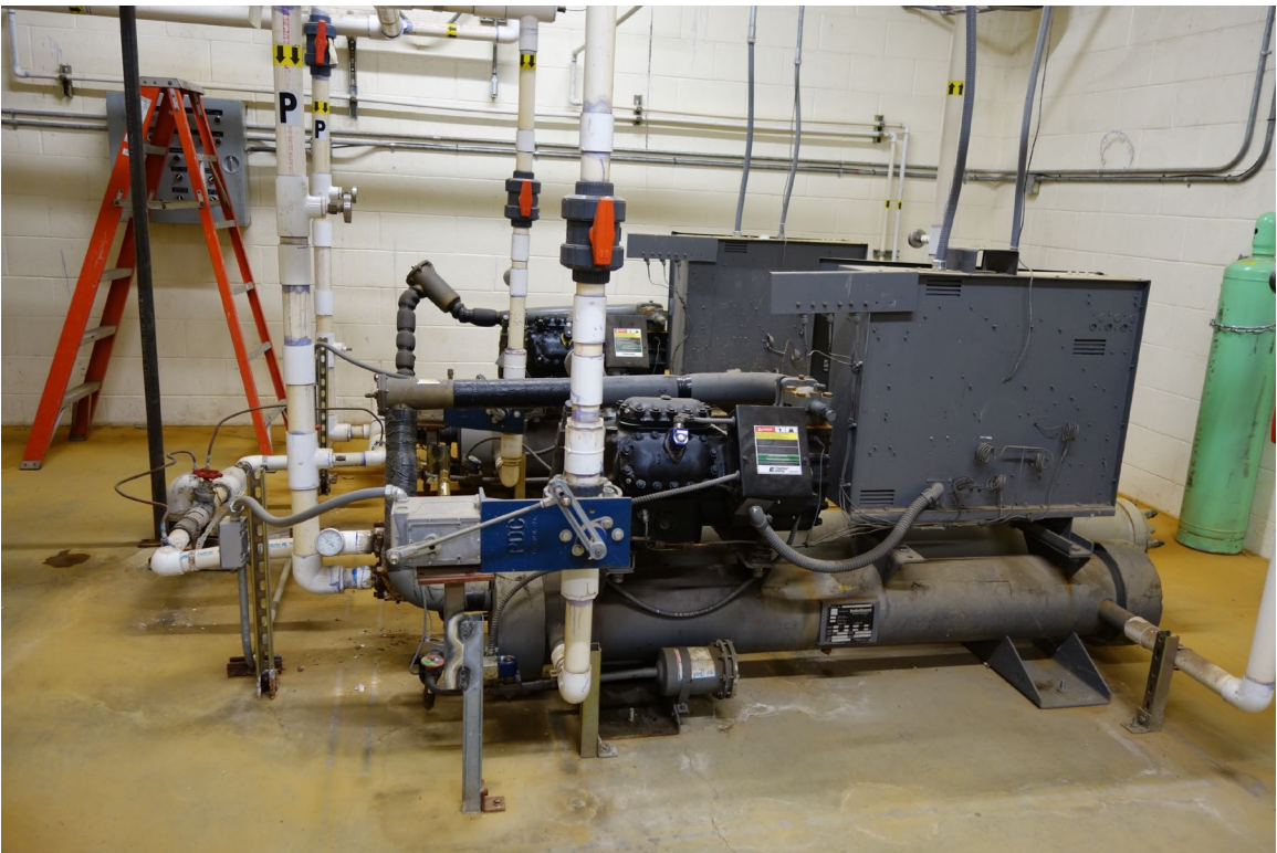
Hatchery Building - Building #1657 Description: Chiller Replacements Needed.
