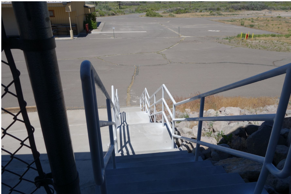
Mason Valley Hatchery - Site #9905 Description: Pavement Cracking West of Raceway.
