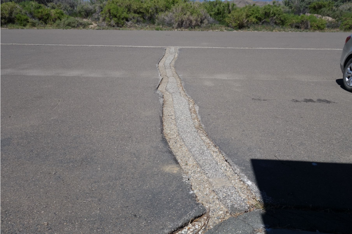
Mason Valley Hatchery - Site #9905 Description: Asphalt Paving Patches Failing.
