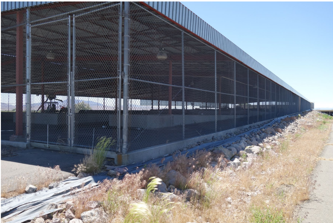
Hatchery Raceway Shelter - Building #2978 Description: Exterior of the Building Needing Rain Gutters.
