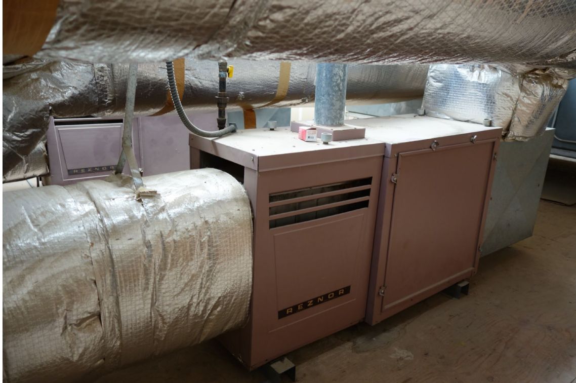
Hatchery Office / Shop - Building #1656 Description: Original HVAC Equipment Needing Replacement.
